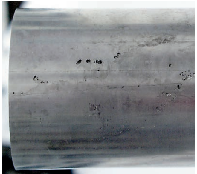
Figure 6:2. Pitting corrosion on the outside of a tube.
