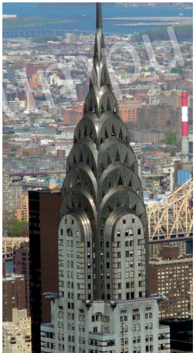
Figure 13:1. Chrysler building in New York erected 1930. During the years, it has only been cleaned twice, with considerable surface deposits accumulation between the cleanings. During its second cleaning in 1995 a few panels near heating exhausts showed some pitting and had to be replaced otherwise in perfect condition.
