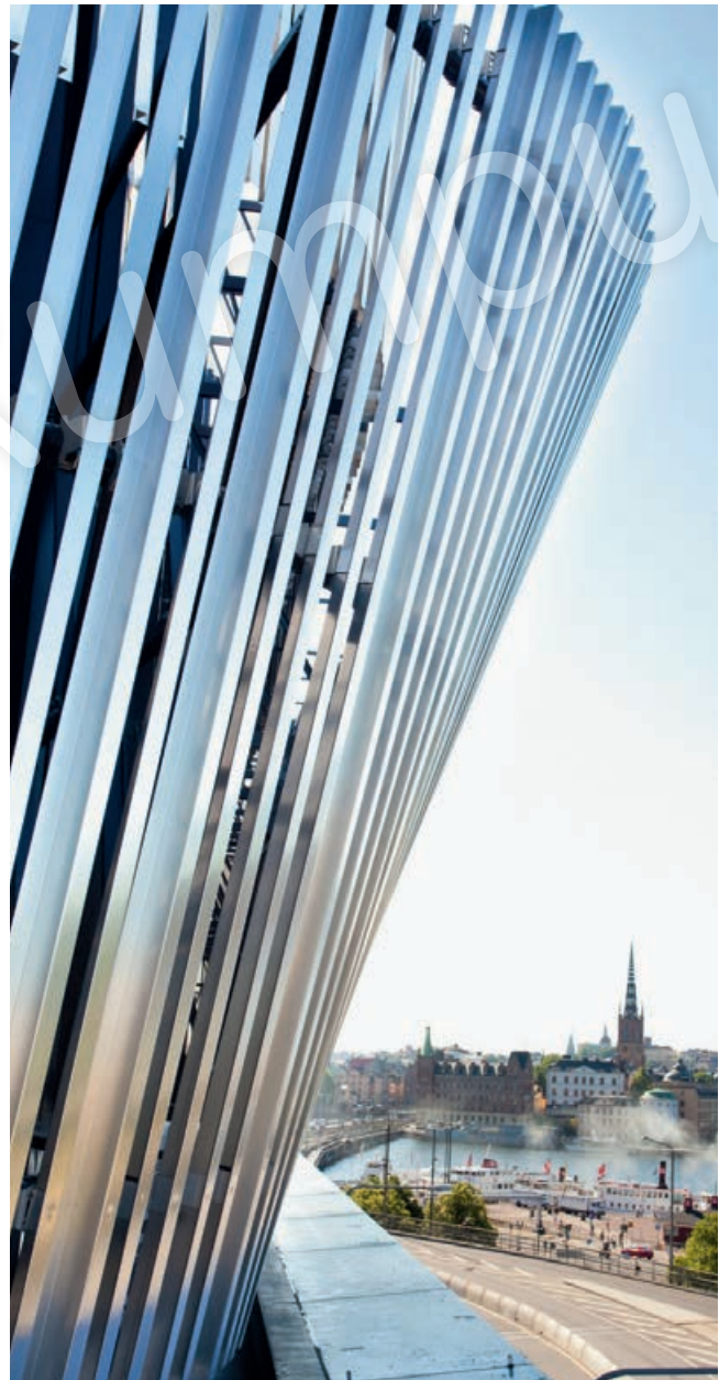
Figure 11:1. Stockholm Waterfront Building, Stockholm, Sweden. Façade made of z-profiles in duplex stainless steel grade 2205.
