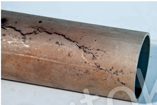
Figure 6:11. Stress corrosion cracking in a stainless steel tube.
