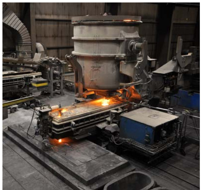
Figure 4:5. Continuous casting. Turret with ladle and tundish, from which the molten steel is led down into the mould by the submerged entry nozzle (SEN).
