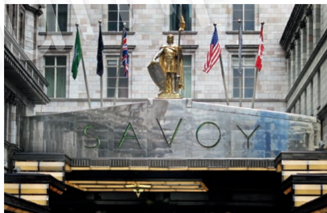
Figure 2:7. Savoy Hotel, London. The sign, made of standard austenitic Cr-Ni type of stainless steel with a polished surface, was completed in 1929.
