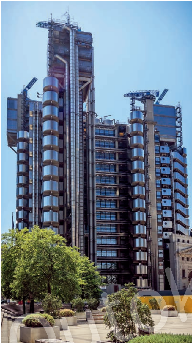
Figure 2:8. Lloyds' Building, London, completed 1986. Cladding in the austenitic Cr-Ni-Mo stainless steel 316 with HyClad® Linen surface finish.
