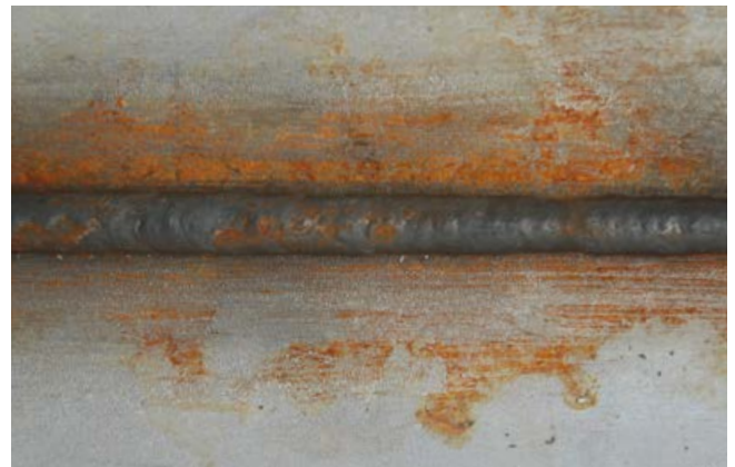
Figure 11:4. Staining caused by iron contamination from mild steel brushing.
