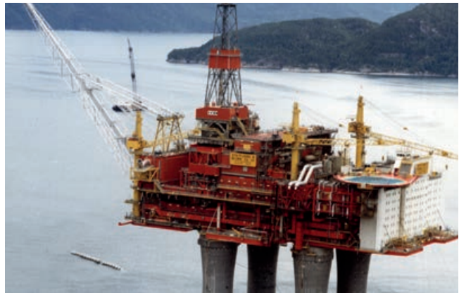
Figure 9:8. Super-austenitic and duplex stainless steels are common materials for different applications on oil platforms.
